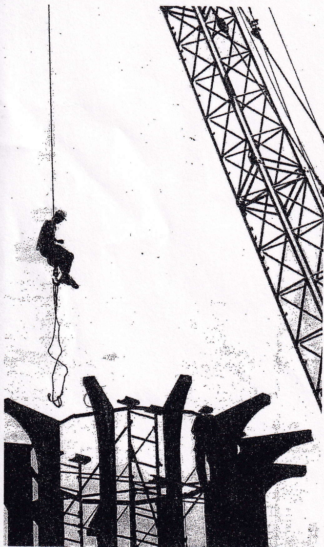
Hitching a ride, a workman checks on the base that will support 1,500 pounds of iron archangels.
